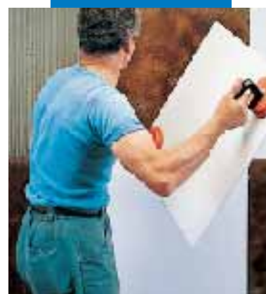
Laying KERAION on a wall
