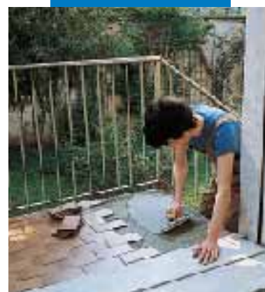
Waterproofing levelling and laying with Kerabond + Isolastic
