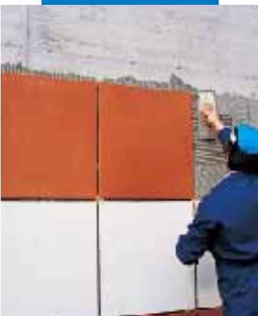
Fixing large size tiles with Kerabond + Isolastic
