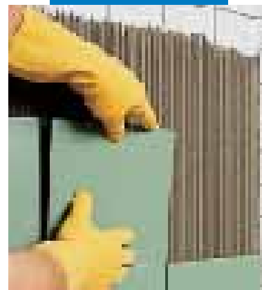
Laying over old tiles
